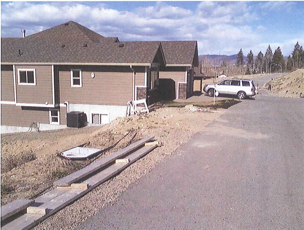
Dwelling at 525 Horn Court
